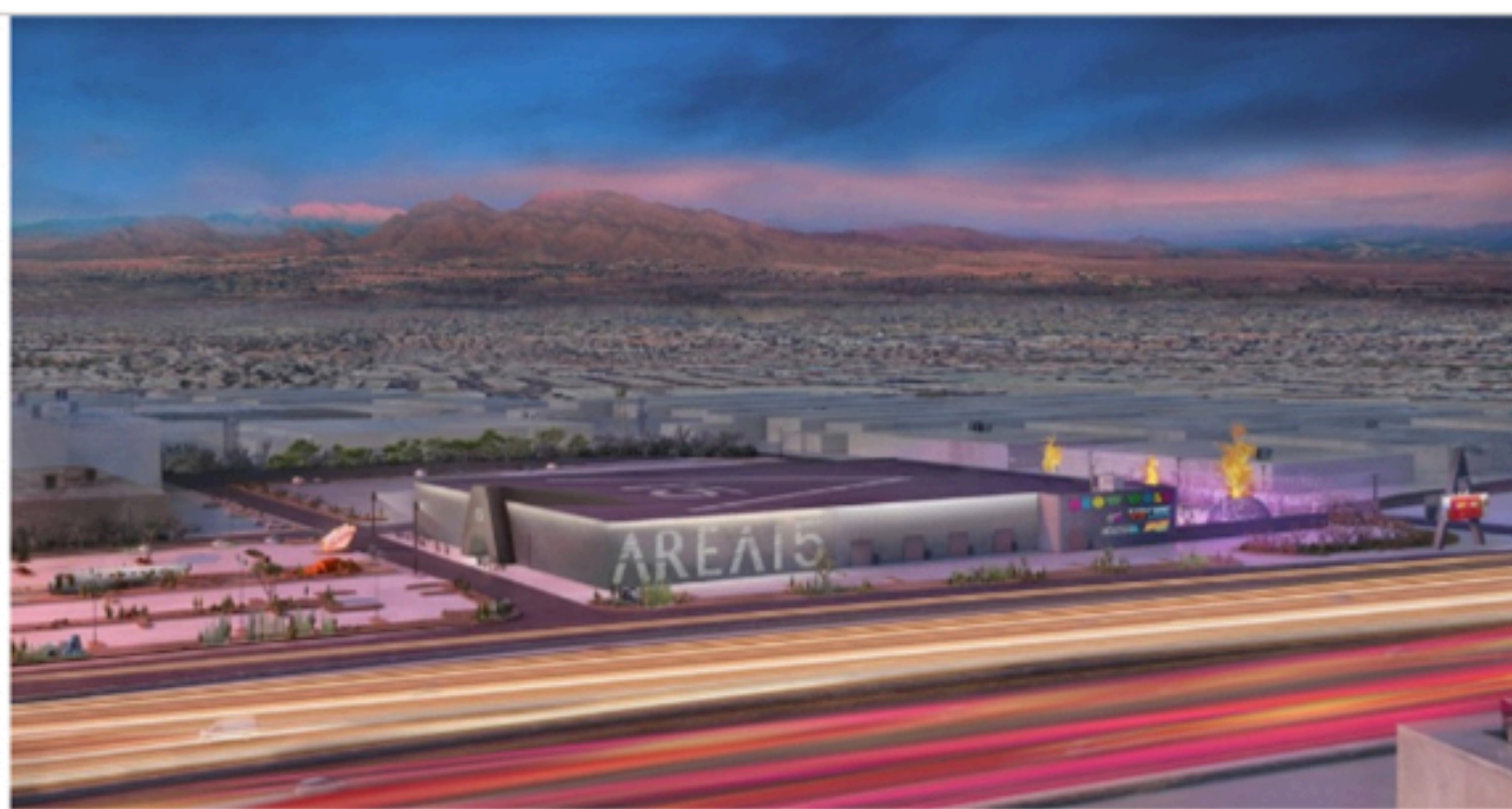
A rendering of AREA15, a wholly reimagined retail, art and entertainment complex opening in Las Vegas late 2019. Credit - A+ (Architecture Plus Information)
